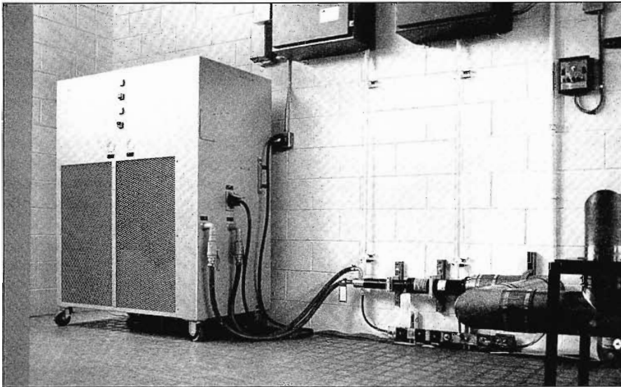
Self-contained, coolant recirculating dummy loads are used. (Visual load above).
